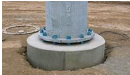
Figure 17 - Drilled shaft foundation
