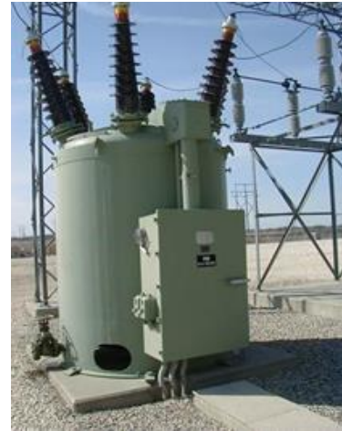
Figure 15 - Pad type foundation
