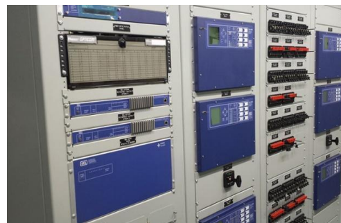
Figure 32 - Relay panel
